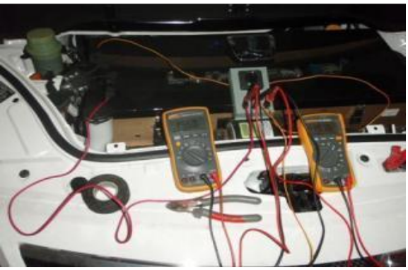
绝缘电阻 Insulation resistance test
