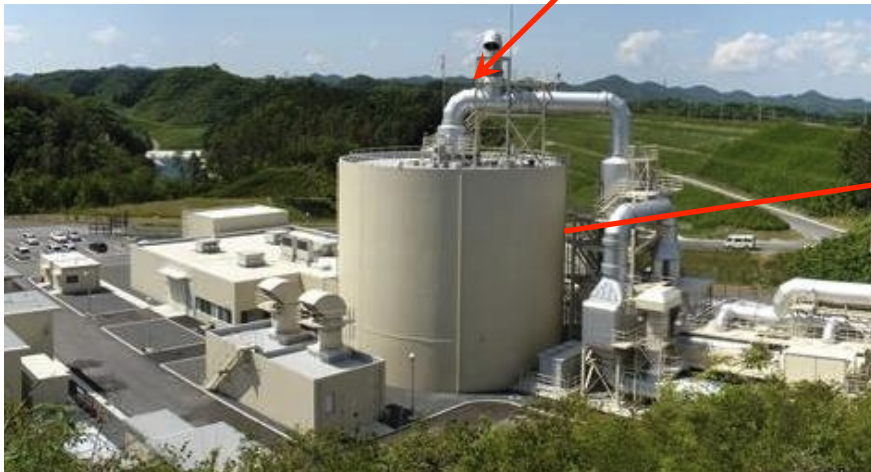
Hy-SEF (Hydrogen and Fuel Cell Vehicle Safety Evaluation Facility)
