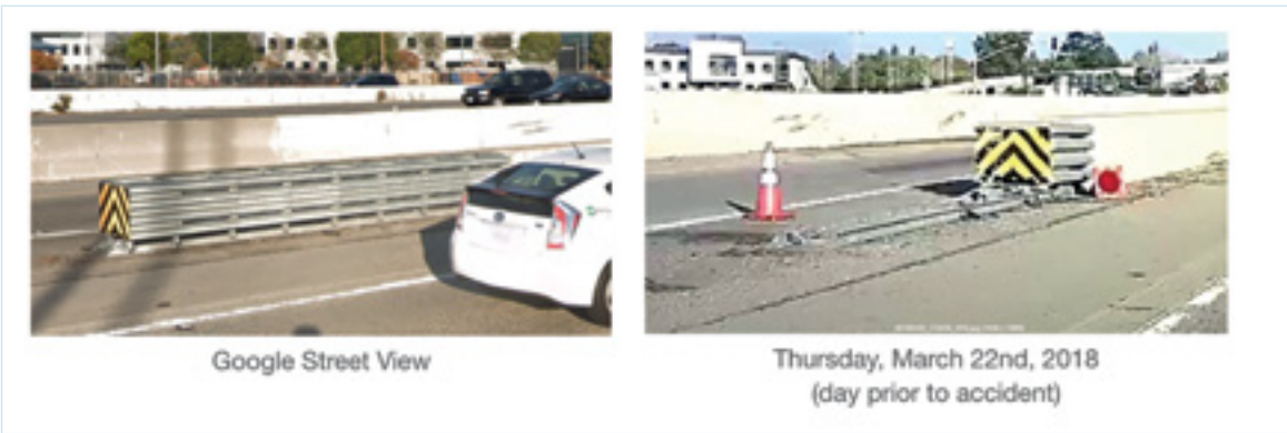
(c) Impact absorber in normal situation and one day before the fatal collision.
