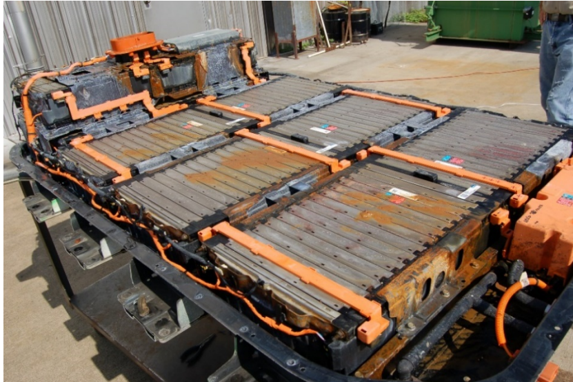
Figure 20. Example pack-level view of battery degradation due to immersion
