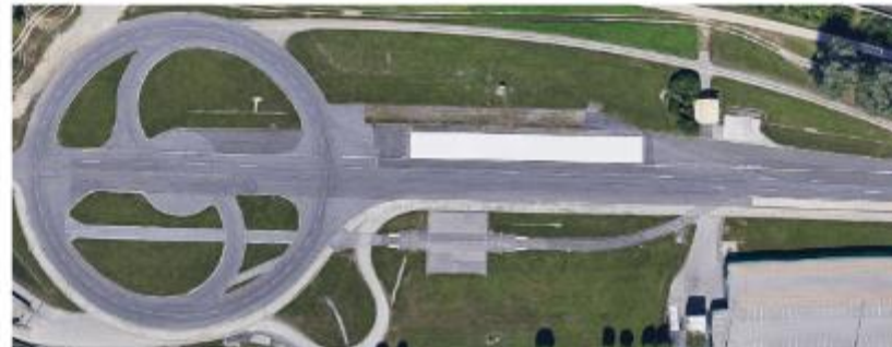
Figure 2: Magna Steyr – Test facility Graz
