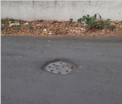
Manhole Below Road Level
