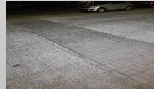
Paved Road Patch
