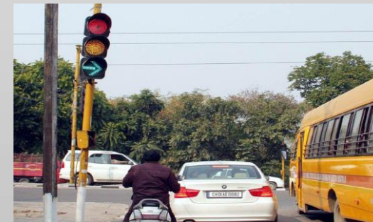
Malfunctioning signal Lights
