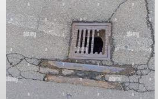
Broken Drainage meshes on road
