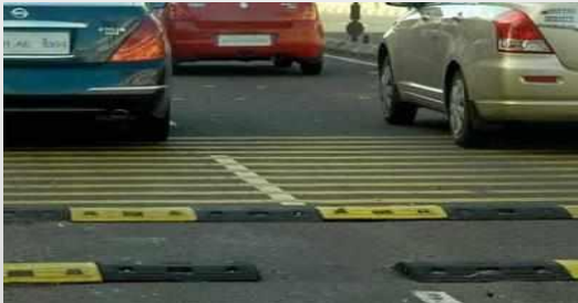
Speed breakers with missing Sections
