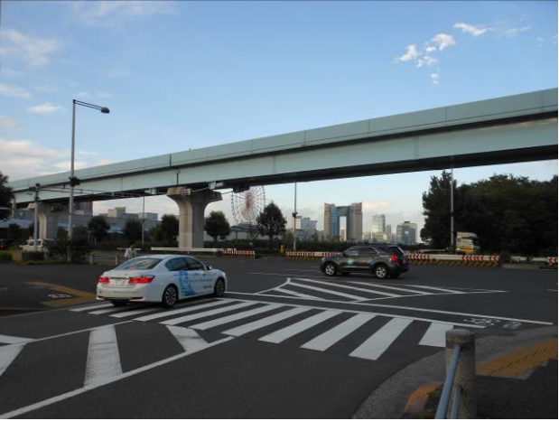
Crossing collision prevention system
