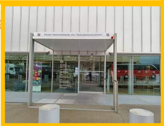
ITU Montbrillant Building Entrance
