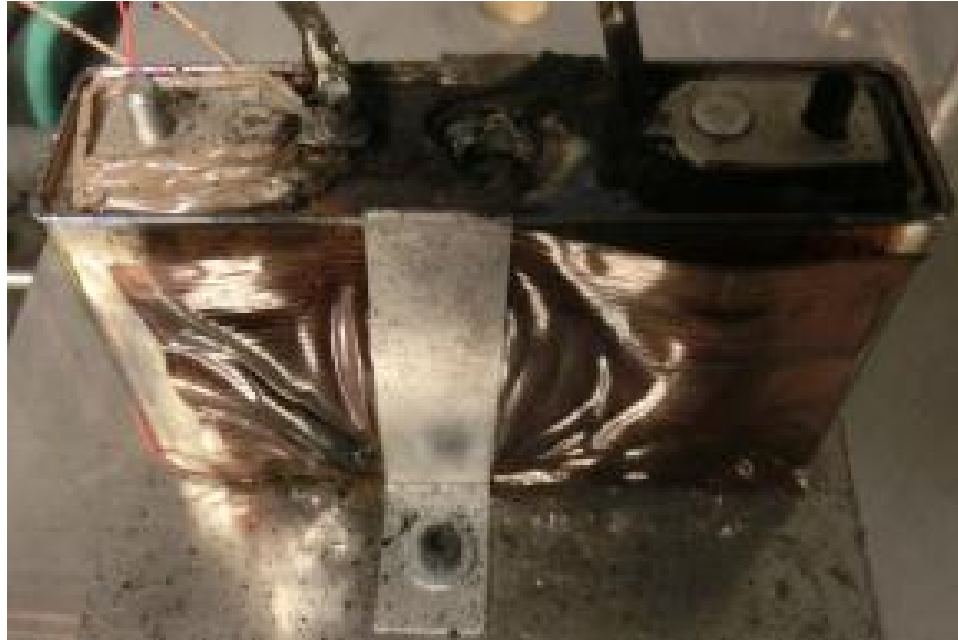
Figure 63 - Prismatic cell after thermal runaway.
