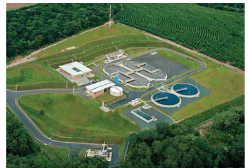
Water Waste Treatment Plant – SESAMM, Mogi Mirim
