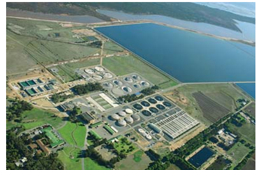
Bolivar Wastewater Treatment Plant
