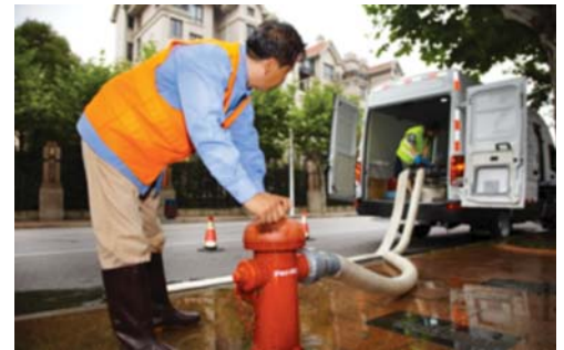
Aquadiag mobile diagnostic truck
