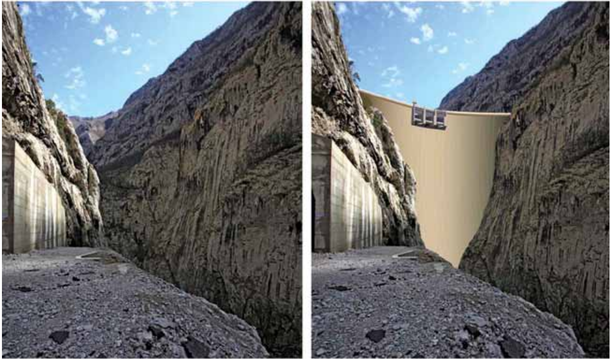
Visual impact of one variant of the Andrijevo dam design on the River Morača, Montenegro.
