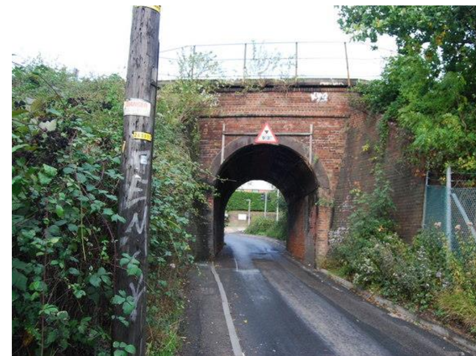
Narrow bridge tunnel, with other oncoming traffic
