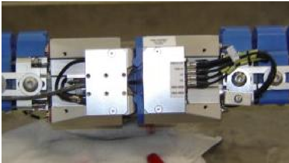
Figure 43 . Right hand side of impact face, lower covers removed
