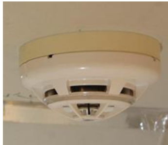
Figure 3. Point smoke/heat detector.
