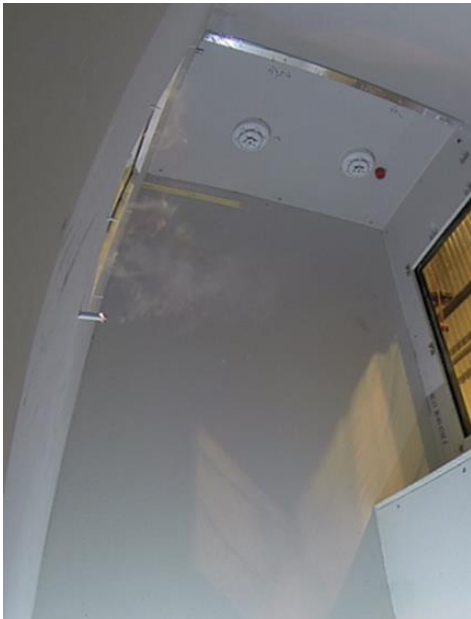
Figure 15. NIST's standard cigarette smoked through toilet compartment wall.
