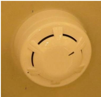
Figure 2. Point smoke detector.
