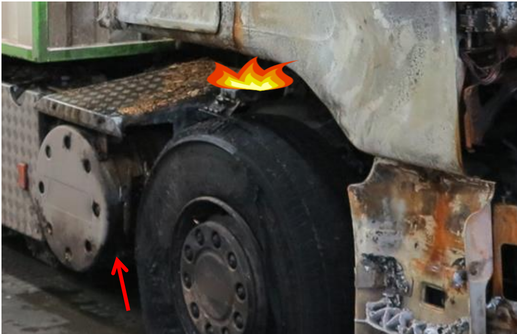
Figure 13 The muffer from Figure 12 is situated in the left in this picture whereas the fire started growing above the tyre, where the mudguard has been consumed by the fire.
