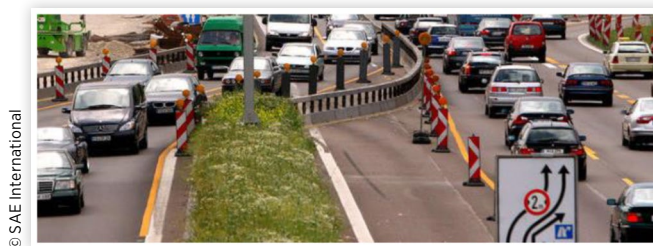
FIGURE 11 Added difficulties in construction zones when the width of the lane changes extremely, allowing only 2 m width of cars.[5]
