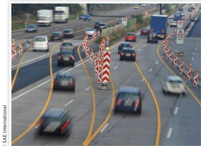
FIGURE 9 Example of a situation where the lanes in a construction zone show some curvature and show reduction in width. [3]
