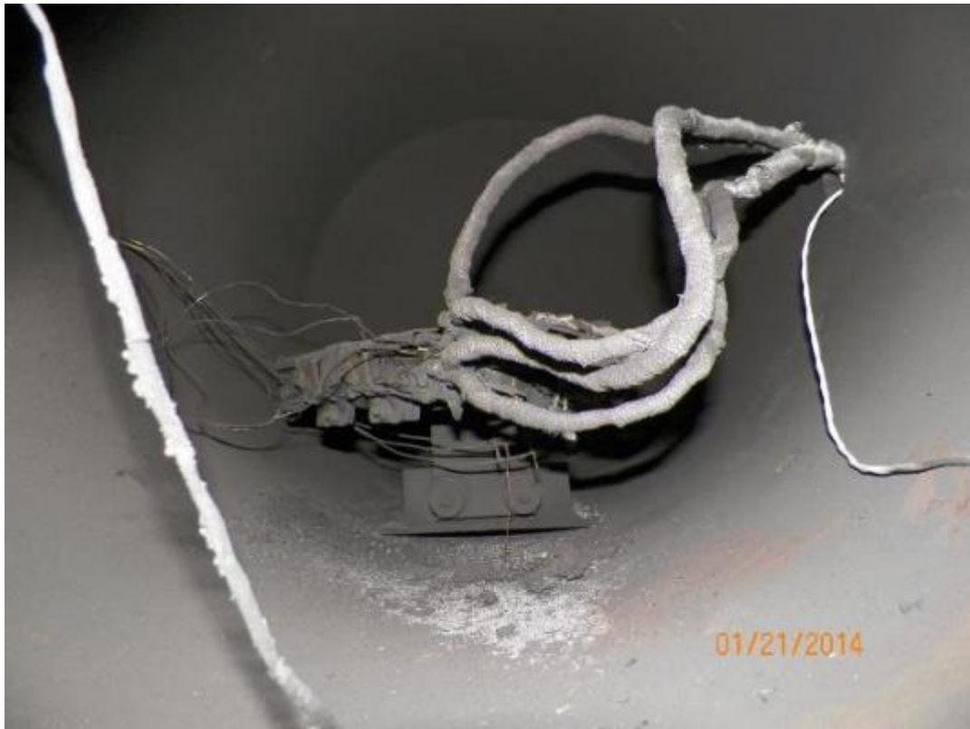
Figure 119 Continuous 32A String Type A Post-Test Fixture (OCICA02)
