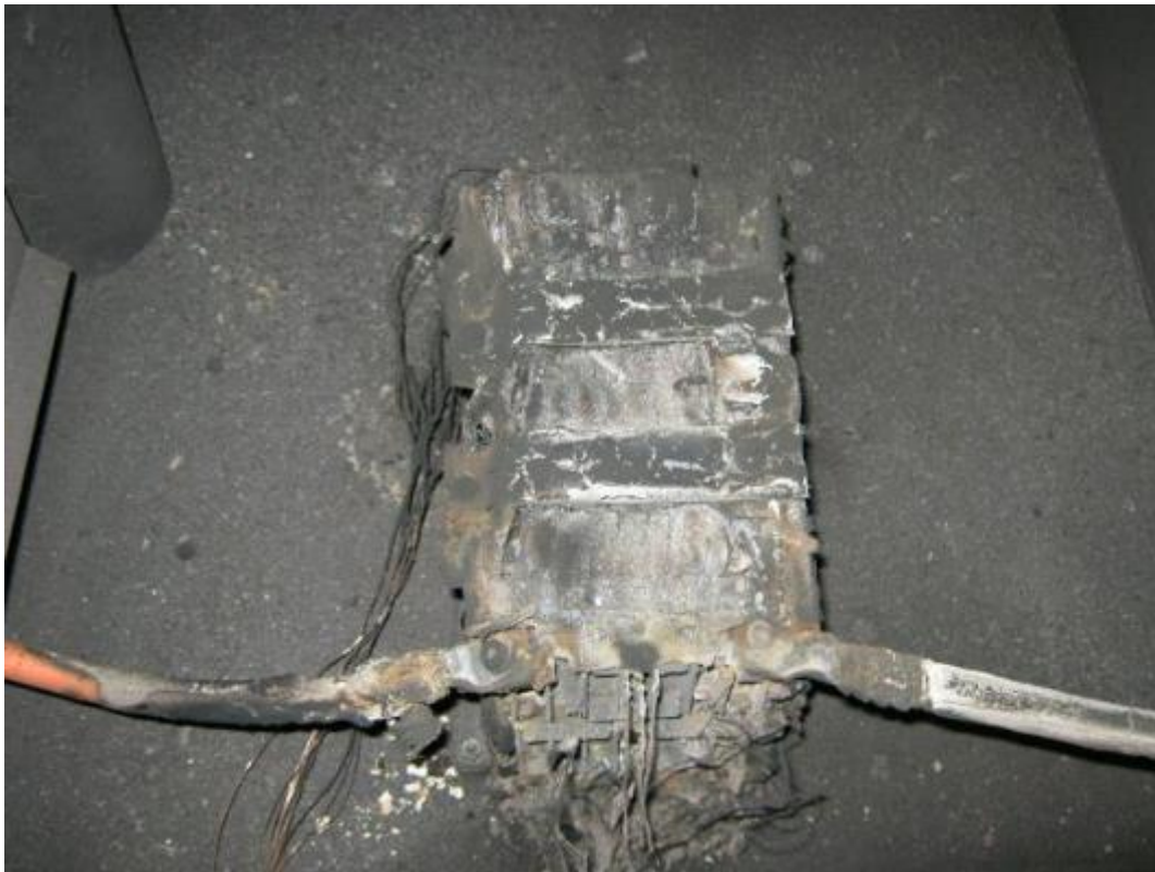
Figure 146 Start/stop 60A Module Type A Post-Test Fixture (OC028)
