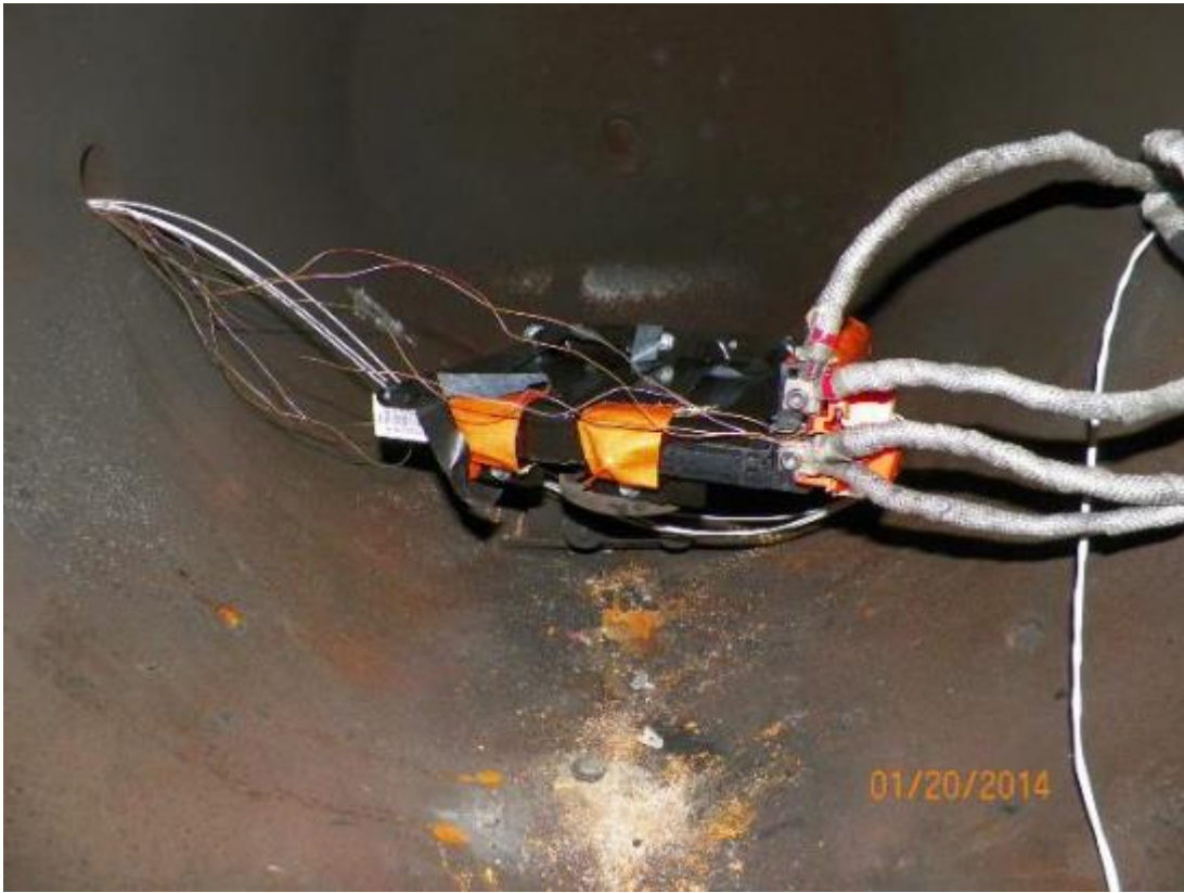
Figure 118 Continuous 32A String Type A Pre-Test Fixture (OCICA02)
