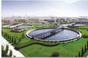
Shandong Ji'nan waste water treatment project
