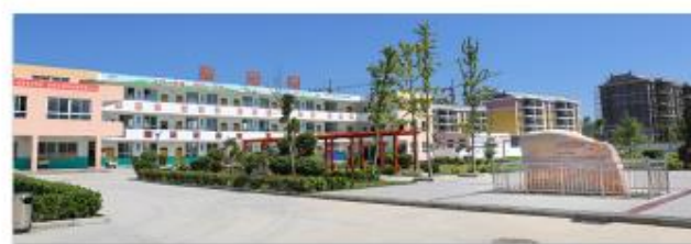
Everbright International True Love School in Dangshan County
