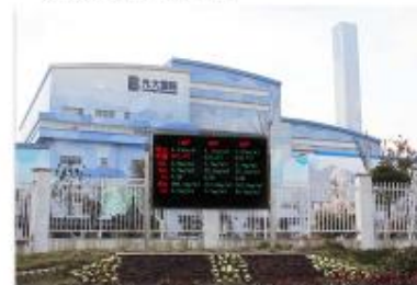
Emission data display board outside WTE Plant
