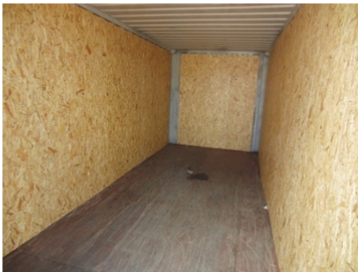
Figure 7.53 Lining a 40-foot container with chipboard panels
